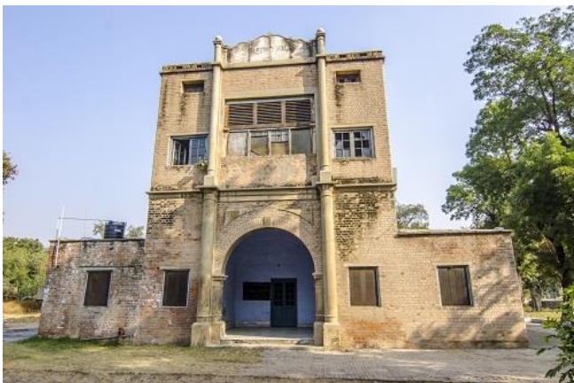
FREEMASONS' HALL, 6A, THE MALL, FEROZEPUR CANTT.
